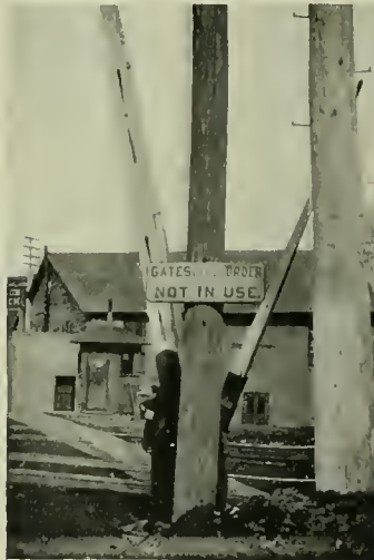
AND THESE ARE CALLED SAFETY GATES.
